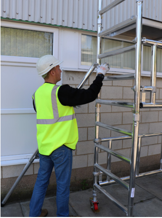
7. Fit 4 stabilizers, one on each upright of the tower. For the 6.1m build use the y250 stabilisers.
