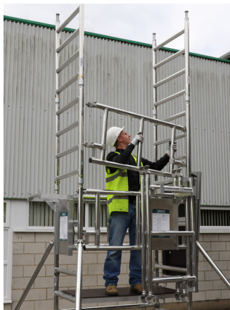
23. Retrieve a side guardrail frame from the front assembly bracket and locate it as shown.
