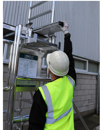
12. Relocate the toeboard assembly from the lower platform to the higher level, ensuring that it is positioned on the plain section of the platform as shown.
