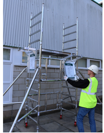
9. Fit the additional assembly bracket on the front of the tower as shown.
