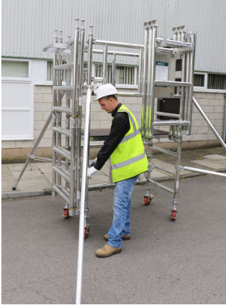
19. Re-Fit 4 stabilizers, one on each upright of the tower if this was not already done.
