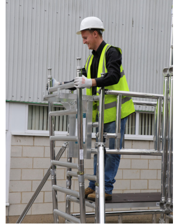
21. Retrieve a set of frames from the side assembly bracket and fit.
