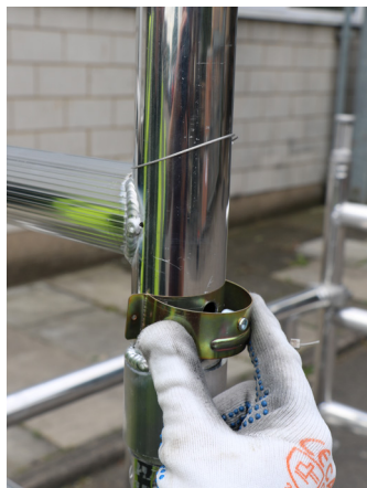
13. Engage interlock clips.
