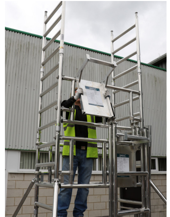
24. Relocate the side "empty" assembly bracket on the front of the tower (top rung of the tallest guardrail frame as shown).
