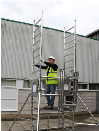
22. Repeat this process for the opposing side, ensuring that all interlock clips are engaged.
