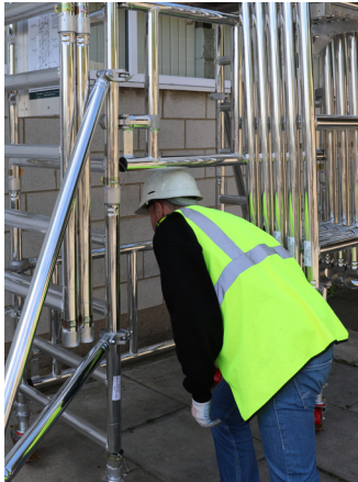
20. Access the platform by passing under the side frame and via the trapdoor platform.
