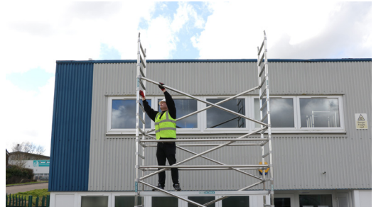
14. fit your additional diagonals to continue the bracing pattern. Running off the rung of your last brace.
