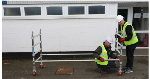
4. Fit 2 horizontal braces to the verticle member of the frames above first rung. Horizontal braces fit on from the inside of the tower facing outwards. (Spigot must be facing inwards)
