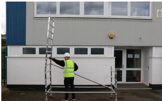
5. Add your next frame ensuring the frame leans inwards and fit 1 diagonal brace from the bottom rung of the 4 rung to the bottom rung of your new frame.
