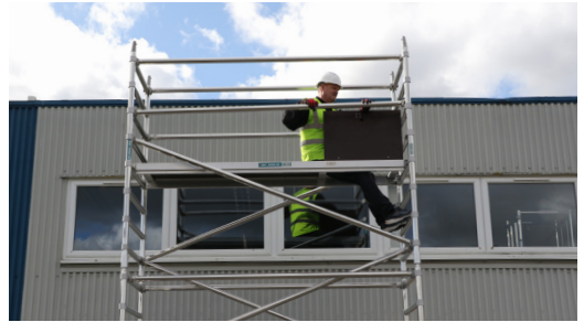
16. From a seated position using the 3T method, fit 4 horizontal braces above the appropriate rungs.
