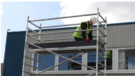
17. Correctly fit toe-boards as shown in the images.
