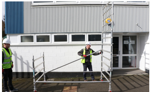
6. Fit 1 diagonal brace from the bottom rung of the 4 rung to the bottom rung of your new frame.
