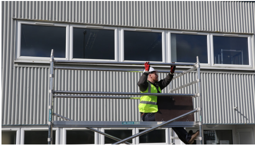
13. From a seated position using the 3T method, fit 4 horizontal braces above the appropriate rungs.
