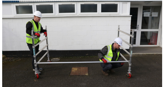
4. Fit 2 horizontal braces to the vertical member of the frames above first rung. Horizontal braces fit on from the inside of the tower facing outwards. (Spigot must be facing inwards)
