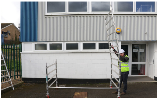
5. Add your next frame ensuring the frame leans inwards
