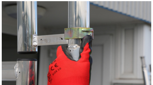
6. After adding frames, always remember to engage all your interlock clips.
