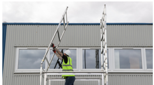
12. Add 4 rung frames ensuring the ladder is continuous. Ensure interlocks are engaged.
