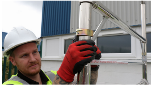
8. After adding frames, always remember to engage all your interlock clips.
