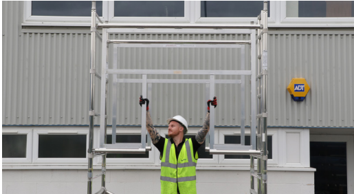
9. Install 4 guardrail braces before accessing the platform. Then fit 2 Advance Guardrail frames, hooks facing outwards ensuring the top hook is located above the top rung.
