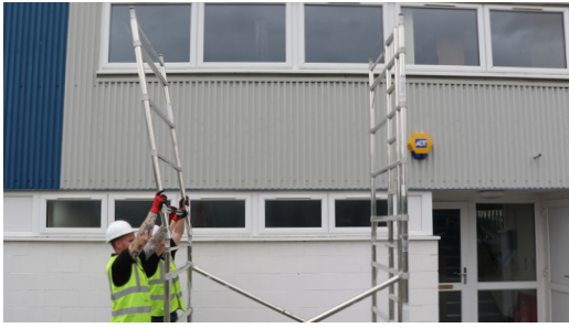
7. Add further frames ensuring the ladder is continuous.
