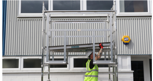
10. Fit 1 trap and 1 plain platform to the 3rd rung down. Making sure the trapdoor is with the ladder section. You can then remove your temporary board and guardrails
