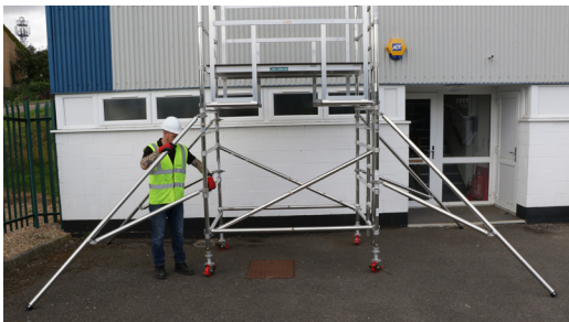
11. Fit 4 stabilisers at earliest opportunity keeping lower arms as horizontal as possible ideally 45 degrees. Stabilisers are fixed onto the frame uprights in each corner by the attached couplers.
