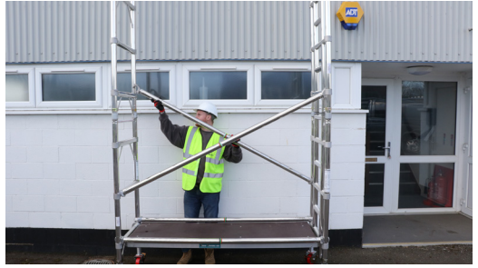
8. Fit 2 more diagonal braces to continue in a regular pattern on the rung above the first platform.
