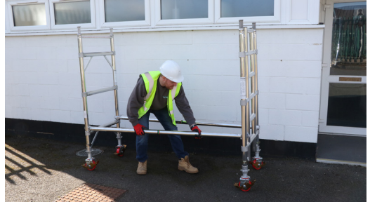
4. Fit 2 horizontal braces to the verticle member of the frames above first rung. Horizontal braces fit on from the inside of the tower facing outwards
