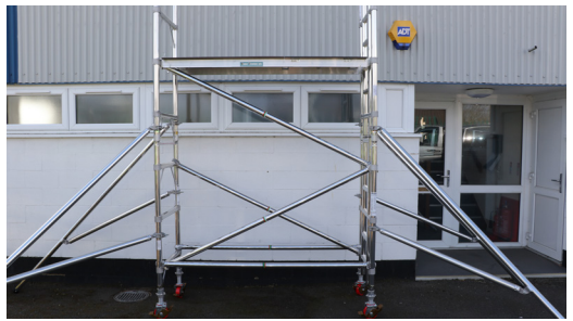
12. Remove temporary platform and the 4 horizontal braces. Relocate 2 diagonal braces from 2nd to 1st rung.
