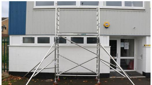
12. Remove temporary platform and the 4 horizontal braces. Relocate the 2 diagonal braces from 3rd to 1st rung.
