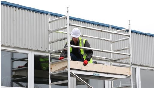
17. Fit toe-boards in correct position
