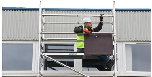
16. From a seated position, using the 3T method, fit 4 horizontal braces above the appropriate rungs to the frame vertices, hooks facing out.
