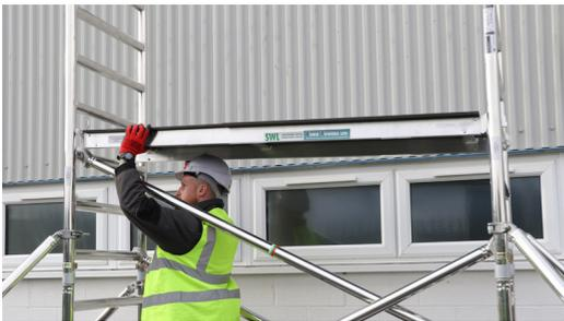
11. From the temporary platform, fit 1 diagonal brace to 3rd rung down and fit trapdoor platform over the hook. Offset platform to oneside and run the diagonal brace away from the trapdoor.
