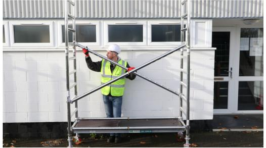
8. Fit 2 more diagonal braces to continue in a regular pattern on the 3rd rung leaving room for your horizontal braces to fit on the upright.
