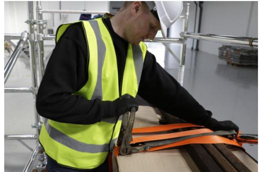
8. Secure the ballast to the platform(s) to avoid accidental removal.
