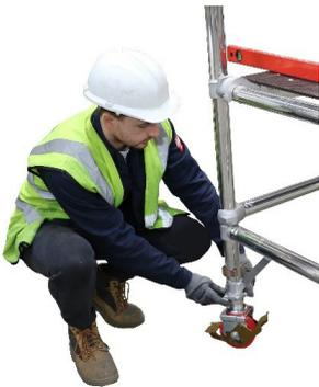
For levelling purposes only, the buttress legs can be adjusted by turning the leg nut as shown.
