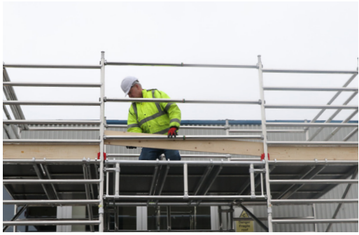
13. Fit your toe-boards to the bridge system as shown in the diagram on page 8 – ref. items 7, 8 & 9
