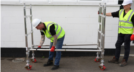
4. Fit 2 horizontal braces to the vertical member of the frames above first rung. Horizontal braces fit on from the inside of the tower facing outwards. (Integral ladder must be on the right hand side)
