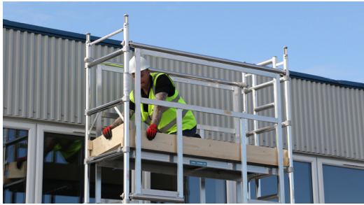
16. Once you have reached the desired working platform height. Correctly fit your Toe-board system as shown.
