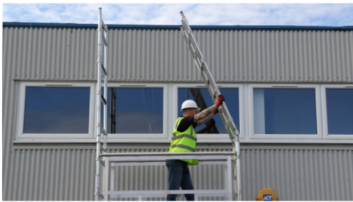
12. Add 4 rung frames ensuring the ladder is continuous. Ensure interlocks are engaged.
