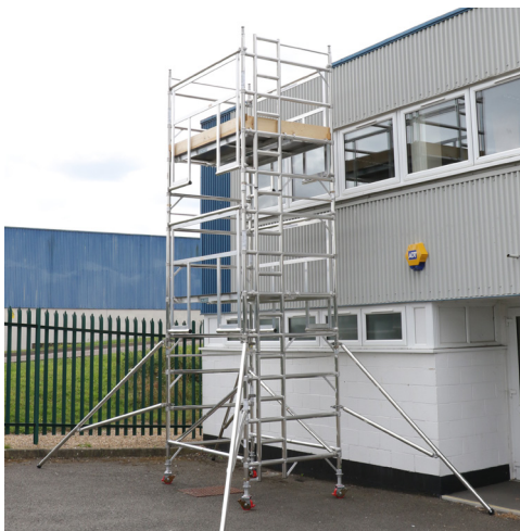
15. Continue erecting tower to final tower height repeating the AGR process (steps 12-14) as illustrated. Always ensure there is side protection to prevent falls. Platforms should be every 2m complete with handrails.
