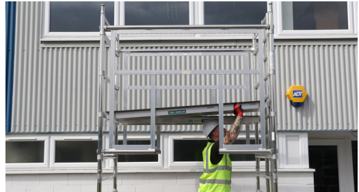
10. Fit 1 trap and 1 plain platform to the 3rd rung down. Making sure the trapdoor is with the ladder section.
