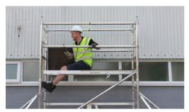
7. Fit 4 horizontal braces to form a guardrail in the seated position using the 3T Method (Through The Trap). Position above the 10th rung and below the 9th using the locator nut.
