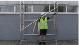
4. Fit one diagonal brace on the front side starting from the 3rd rung to the 7th.
