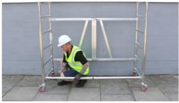
2. Fit one horizontal brace to the vertical above the first rung of the unit, on the opposite side of the folding gate (*Front side*).
