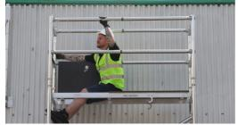
11. Fit 4 horizontal braces to form a guardrail in the seated position using the 3T Method. Position above the rungs of your guardrail frames.
