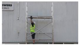
10. Fit your next trapdoor platform to the 3rd rung down from the top. This will be the top rung of your TT4F.
