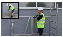
1. Ensure all castors are firmly fitted to the folding frame. Then open folding frame and engage toggle clamps.
