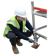
For levelling purposes only, the legs can be adjusted by turning the leg nut as shown.
