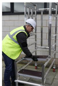
Fit the step platforms on the 1st and 2nd rung as seen above.
