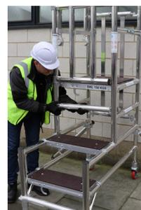
Add the additional brace below the platform. For a stepfold 2 you should now have 2 ribbed braces below the working platform.
