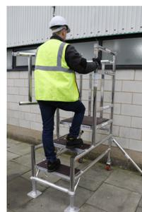
Ascend to the platform using the step platforms and ribbed brace.
