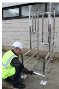
Fit a ribbed brace above the lowest collar as shown.
