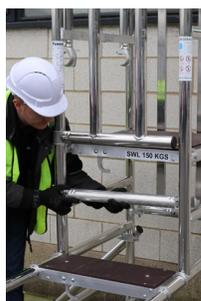
When building the Stepfold 2 add a ribbed brace below the platform.
