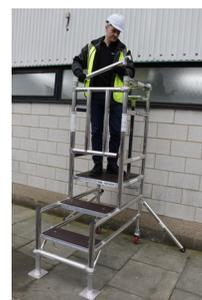
Once the platform is accessed, close the gate behind you; ensure that the clips are engaged and fit the 2 guardrail braces.
