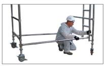
Fit in 2 horizontal braces to the vertical member of the frames, as low as possible, below the 1st rung. All horizontal braces fit on from inside the tower facing out.
