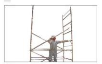
Klik in diagonal braces to continue in a regular pattern. Double Width towers always have diagonal braces either side of the tower opposing each other as illustrated.
