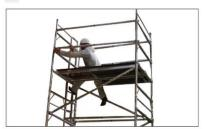
Dismantling is the reverse except when dismantling the handrails, Unclip the four end hooks and from the sitting position remove the handrails. Do not remove the handrails whilst standing on the platform, this would leave you at risk.
