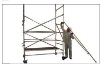
Secure stabilisers as soon as possible to increase tower stability. Check tower kit list to ensure the correct stabilizers are fitted.
