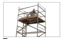
When handrails have been correctly fitted, fit toeboards.
