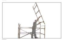
To add further frames, stand on platform ensuring the ladder frames are in line.
