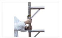
After adding frame always engage interlock clips
