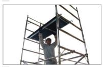
Remove plain platform from the bottom and reposition as shown.
