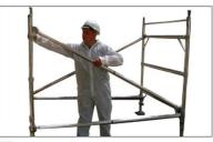
Klik in diagonal braces, starting at the bottom rung. Braces should be added in a continuous patter. When fitting a full intermediate work platform it is permissible to interrupt the continuous pattern.
