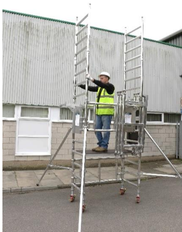
22. Repeat this process for the opposing side, ensuring that all interlock clips are engaged.
