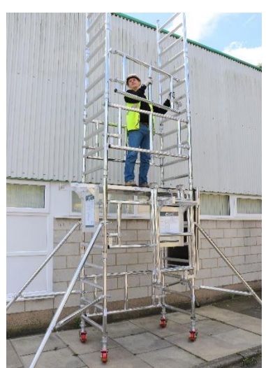
20. Fit 1 side guardrail the 3 rd rung above the existing as shown.
