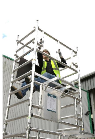
28. Fit 2 guardrail frames, with the top hook (facing outwards) set above the top rung of the frame.
