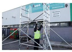
7. Fit a trapdoor platform to the 4<sup>th</sup> rung, trapdoor to the ladder end. **Note:** Platforms are positioned every 4 rungs
