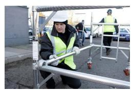
Fit another horizontal brace on the ladder side of the frames face down onto the 1st rung.
