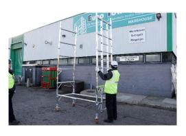
Fit the next set of frames onto the base, ladder frames run continuously. Note: see kitting page for frame lists.
