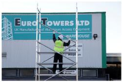
10. Add diagonal braces continuing the pattern from the previously fitted braces.
