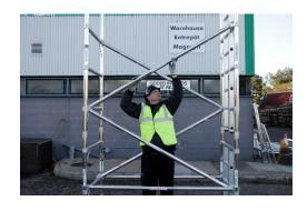
5. Add 4 diagonal braces from the  $1^{st}$  to  $3^{rd}$  and  $3^{rd}$  to  $5^{th}$  rungs as shown, level the tower using a spirit level as a guide. The scaffold must be vertical in both planes within an inclination of 1%.
