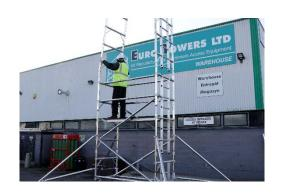
9. Standing on the platform, add a set of 4 rung frames, ladders run in a continuous pattern.
