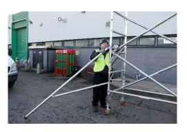
6. Fit the 4 stabilizers supplied with your tower. **Note:** Always fit 4 stabilizers unless building in a corner, inner stabilizers fit parallel to a wall. See kit list for correct size required to build your tower.
