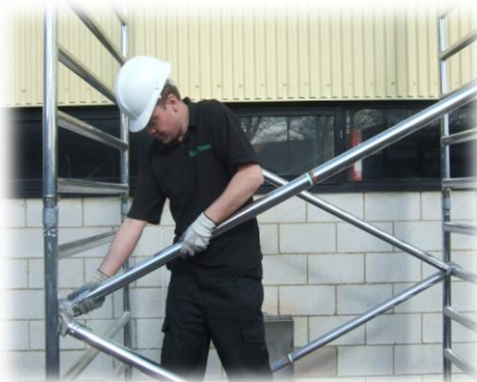
Lock Castors and level the tower, Insert diagonal braces in a regular pattern opposing each other as illustrated.
