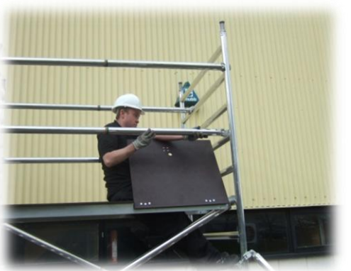
From the sitting position, through the trapdoor (3T Method) Fit horizontal braces as mid rails and guardrails to the vertical member, Hooks facing outwards.
