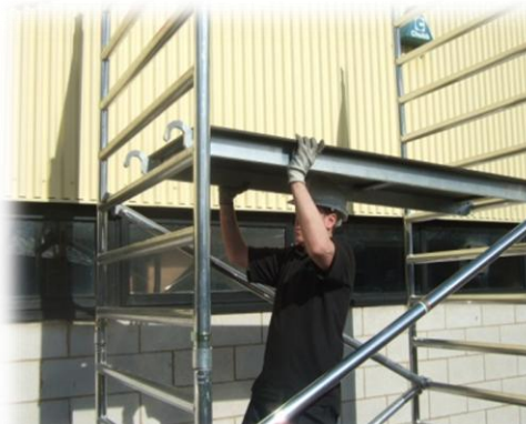
Put platform on the 9 th rung.
