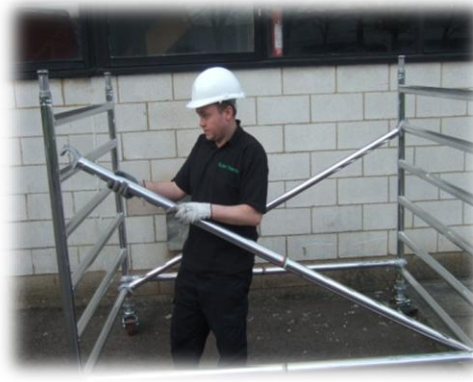
Fit in 2 diagonal braces, starting at the bottom rung – on opposing sides.
