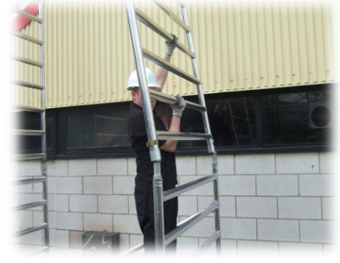
Add 2 frames, after adding any frames always engage the interlock clips
