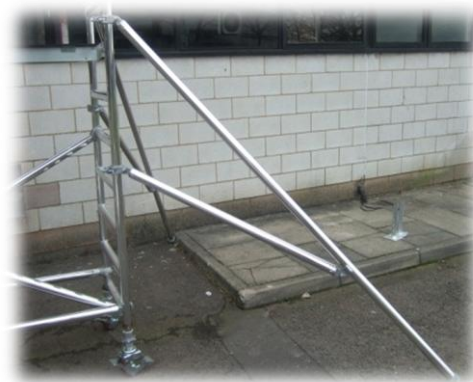
Fit stabilizers at this point
