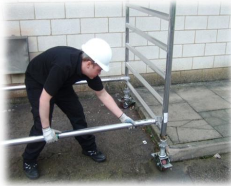
Fit 2 horizontal braces to the vertical member of the frame as low down as possible.
