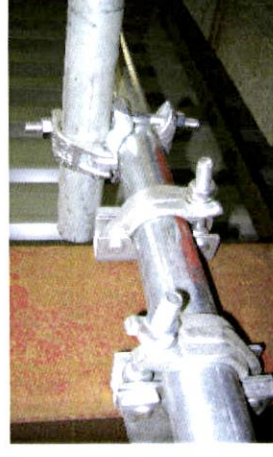
Fig. 5 – Girder Couplers (vertical)
