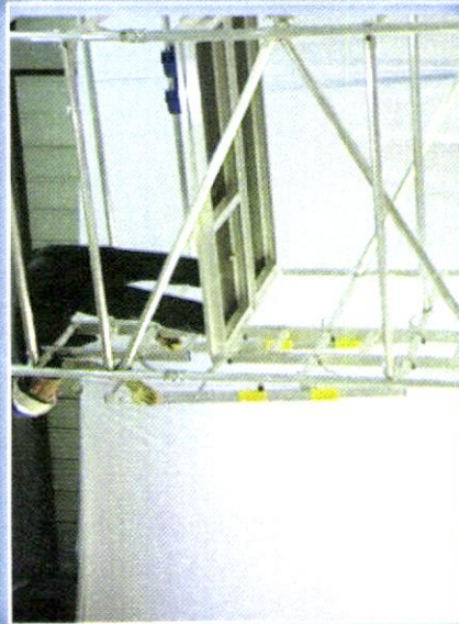
16. Aluguard frame can be either connected to the outside of the lower frame or removed...
