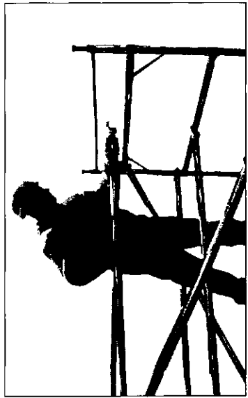
7 Fit four handrail braces, two on outside and two on mid rung of frame as shown, on lower levels these may not be required.
