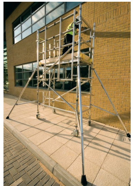
Stabilisers or outriggers must be deployed to their full extent and the weight needs to be properly supported.
