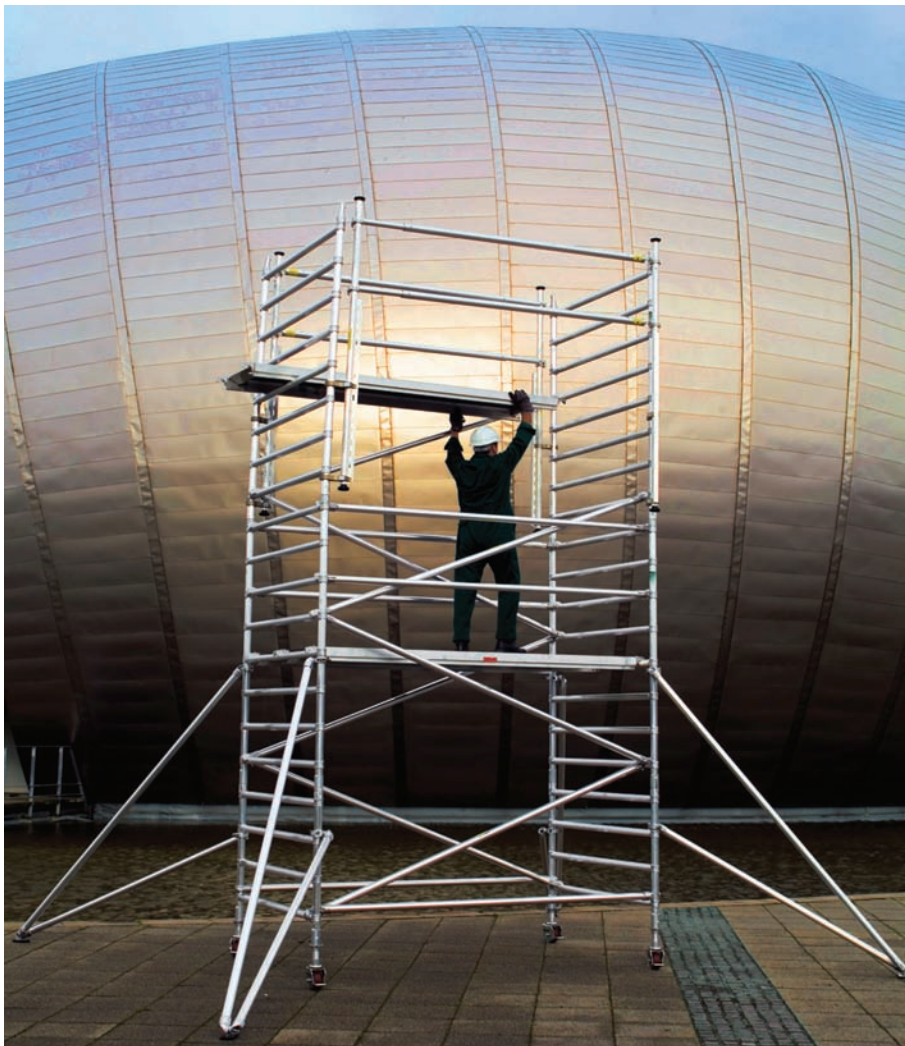
Mobile access towers provide a safe means of gaining access to work at height.
